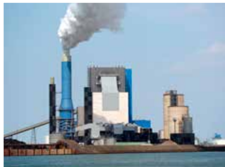
Engie kolencentrale Rotterdam (sinds 2015)
